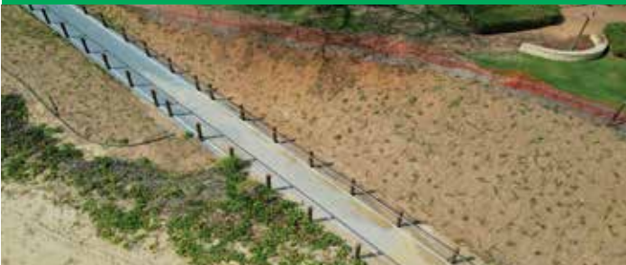
1. Bargara Beach Project
