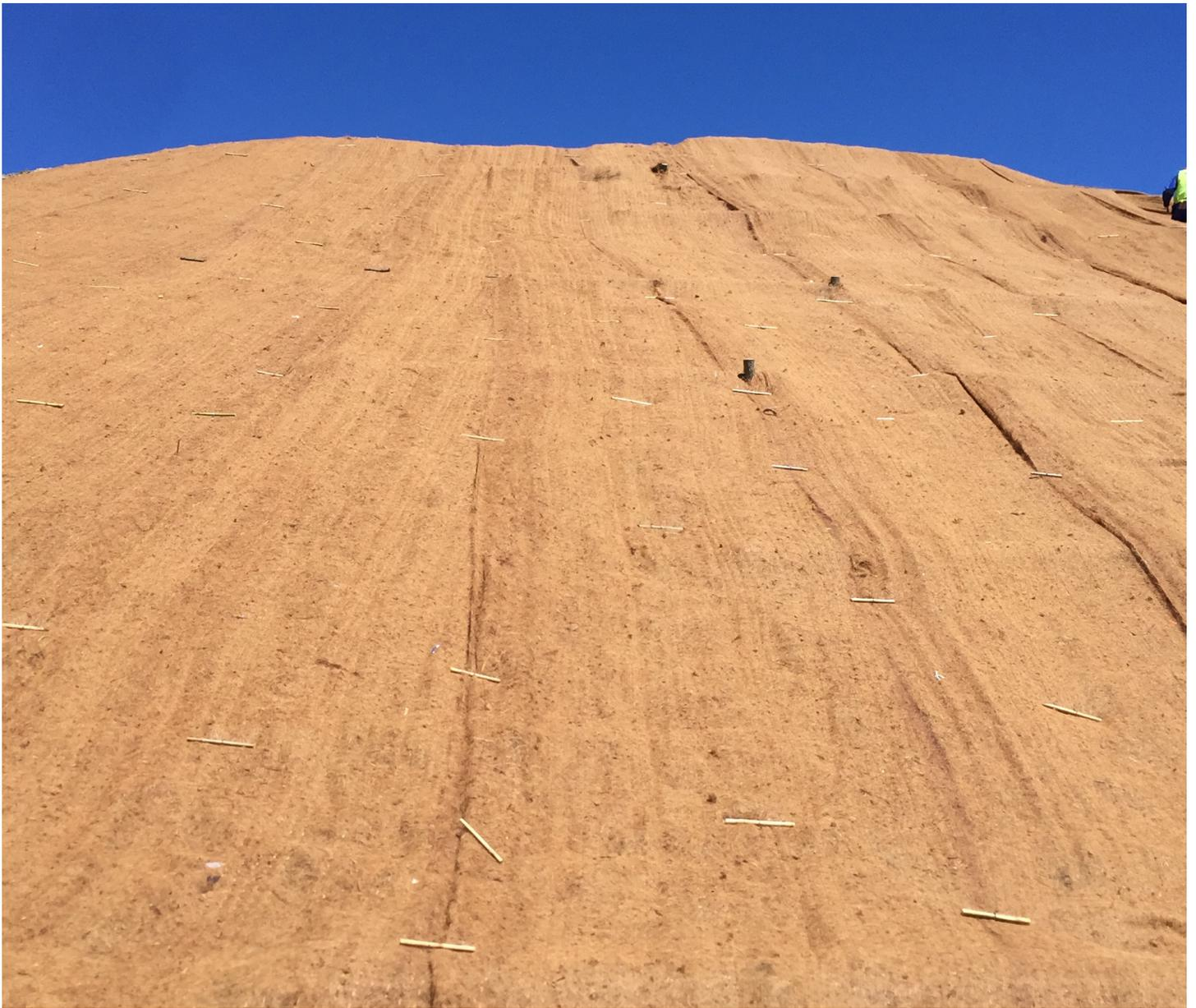
The wide range of EnviroBlanket™ cater for an extensive variety of different soil types, slopes, and gradients. Depending on the type of fibre and thickness/weight, they have a life duration of approx. 1-5 years, in which time the vegetation cover will have taken over the task of erosion control.
