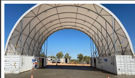
THIESS MT ISA - ANTHILL MINE Heavy Vehicle Workshop Slab
