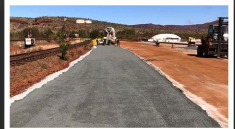
RioTinto PILBARA Access Road and Rail Loading Facility
