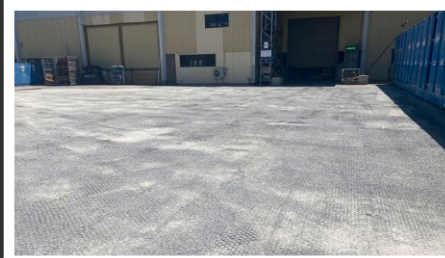
GLENCORE COLLINSVILLE COAL Warehouse & Hardstands
