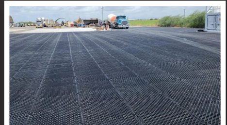
SBS Heavy Haulage MACKAY QLD 6,000m 2 Concrete Hardstand
