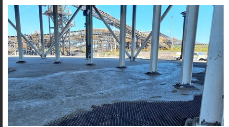
Coronado CURRAGH MINE Concrete Pavements around the fixed plant
