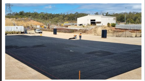
RioTinto BOYNE SMELTER Laydown Area + Hardstands
