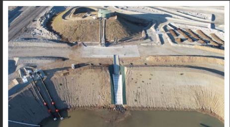
GLENCORE MANGOOLA COAL Water Truck Fill Point & all weather Access Roads
