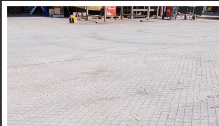
MACKELLAR BLACKWATER QLD 7,600m 2 Concrete Workshop Pavement
