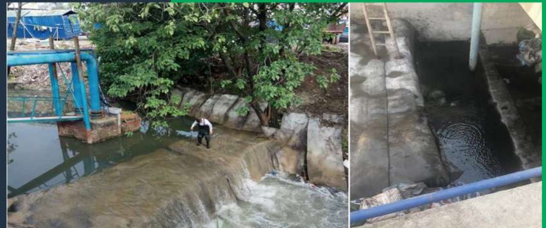
Sewage treatment plant
