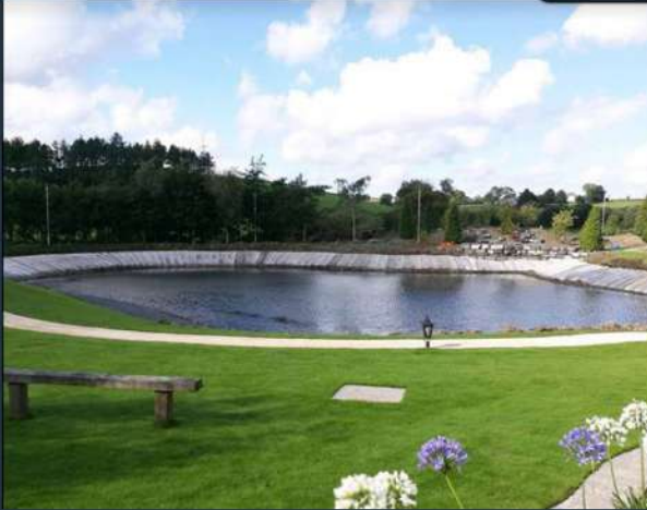
Bank erosion project
