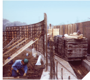
Curved Wall Forms using Steel-Ply
